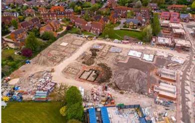
"After completing the main infrastructure, road and drainage works for the Wantage site, we then undertook the groundworks for St Modwen Homes on the 1B Parcel. Works consisted of groundworks for 101 houses and flats with associated infrastructure. The units comprise traditional strip foundations with brickwork and block beam floors. As a valued client, we hope to have many more schemes for St Modwen Homes in the future."
